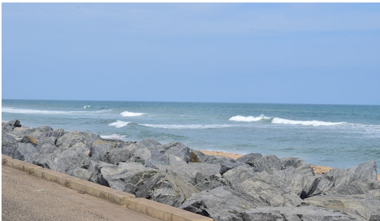
Figure 6: An image of the coastal defense structure along the Akplowotorkor-Dzita stretch
